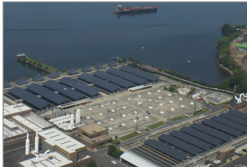
Camden Solar Center 1.8 MW | Camden, NJ PPA: Camden County MUA
