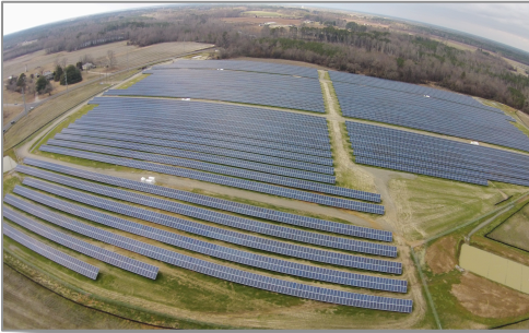
Boseman Solar Center 5 MW | Nash County, NC PPA: NCEMPA
