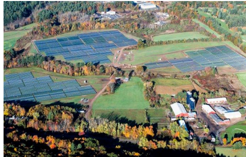
Somers Solar Center 5 MW | Somers, CT PPA: CT Light & Power
